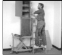
Positioning cabinets in construction.
